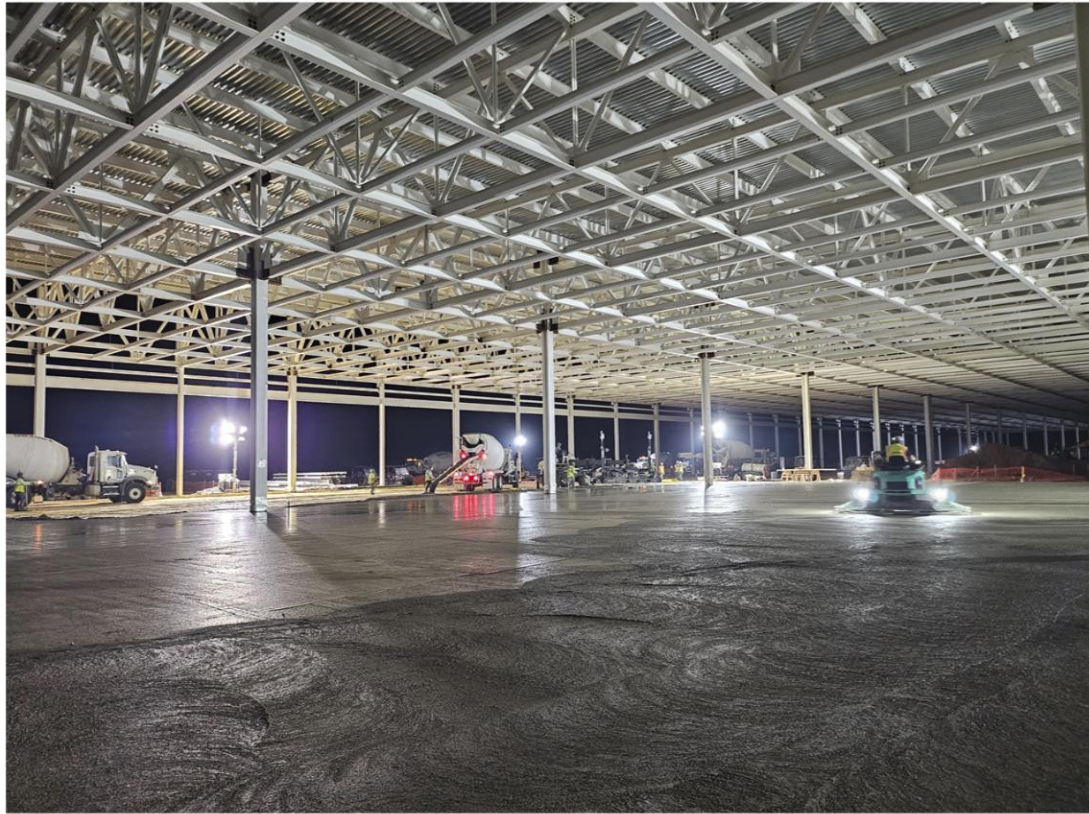
G2_AUSTIN CONSTRUCTION IN JULY 2026
